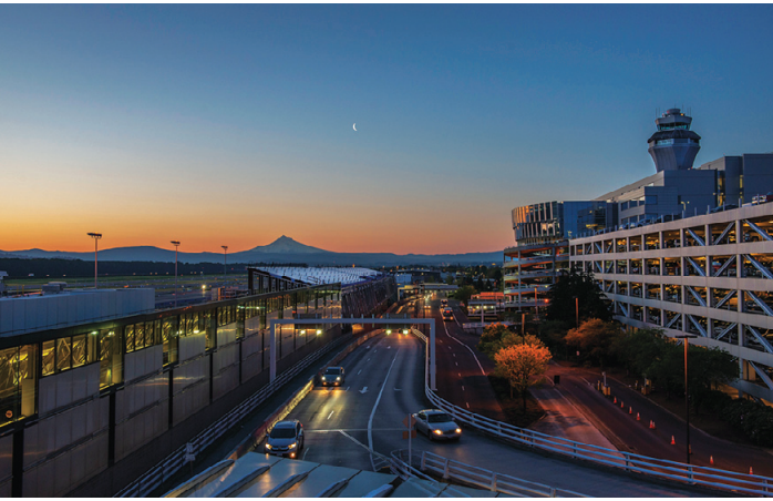
Aside from modernizing its facilities, Portland International Airport (PDX) is also expanding its network around the world. In March, Delta Air Lines will launch a nonstop flight to Tokyo's Haneda Airport in time for the Olympics.
